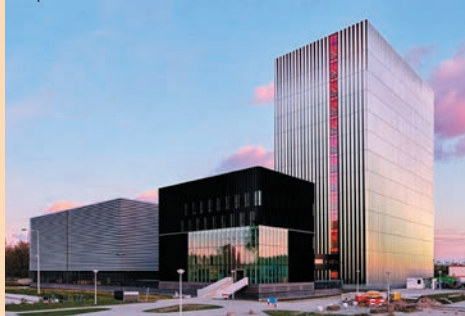
Equinix AM4 Data Center in Amsterdam.
